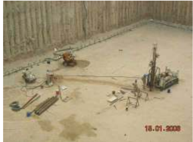
Soil test being undertaken for Wind Tower I
