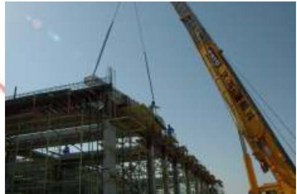
Tohid Iranian School, Dubai, under construction
