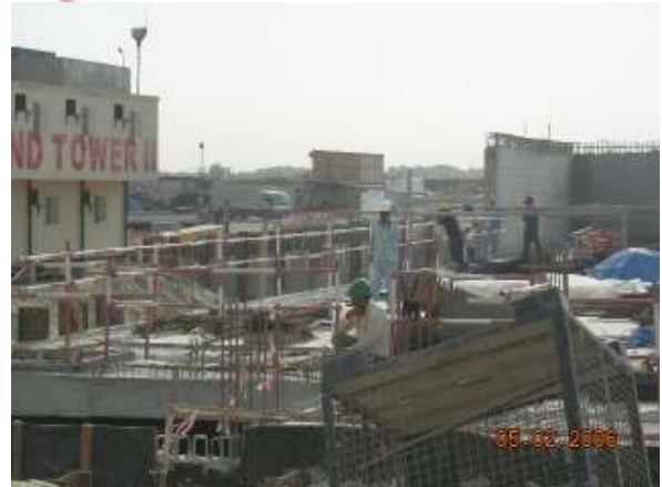
Outdoor Parking at Wind Tower II's construction site
