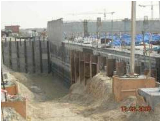
Back Filling at Wind Towers' Outdoor Parking Area
