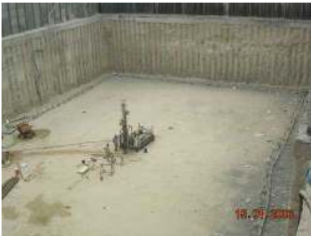
Swiss Boring Undertaking Soil Test for Wind Tower I
