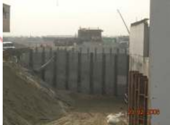
Water Proofing at Wind Towers Construction Site
