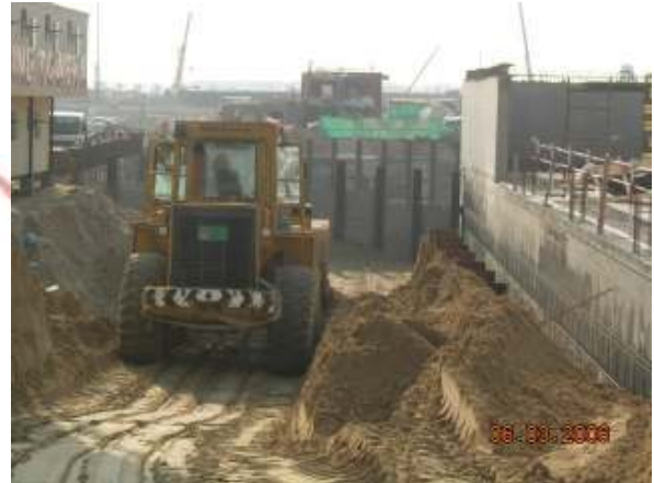
Wind Tower Construction Site
