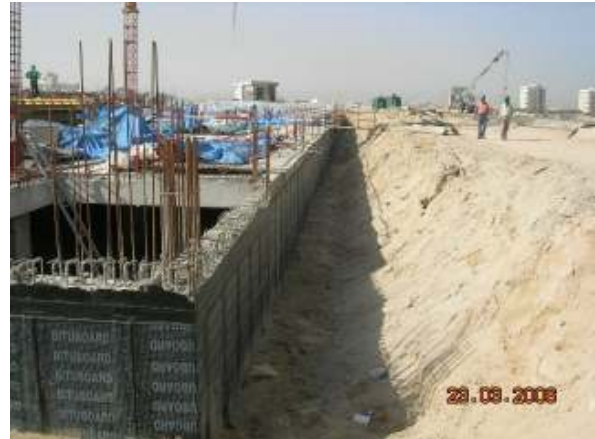
Back-filling at Wind Tower's construction site
