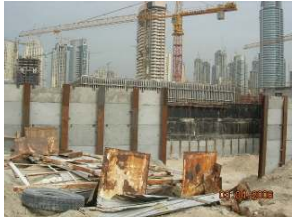
Wind Tower II construction site
