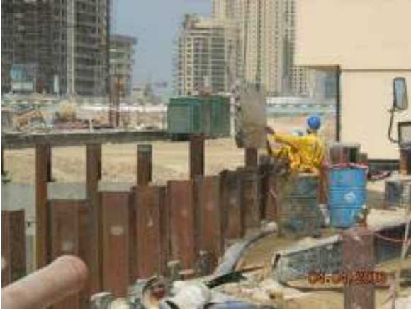
Concrete Panel Excavation
