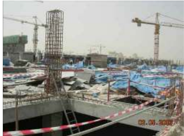
Reinforcement for Parking Area
