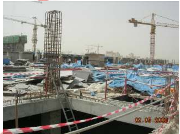
Construction for Parking Area
