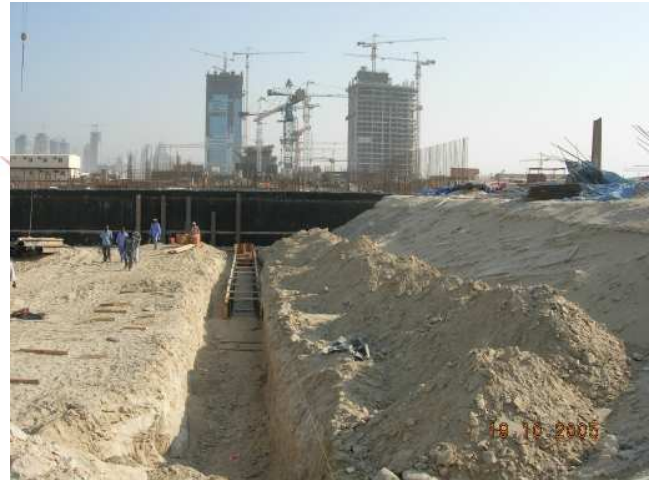
Construction site for Wind Tower II
