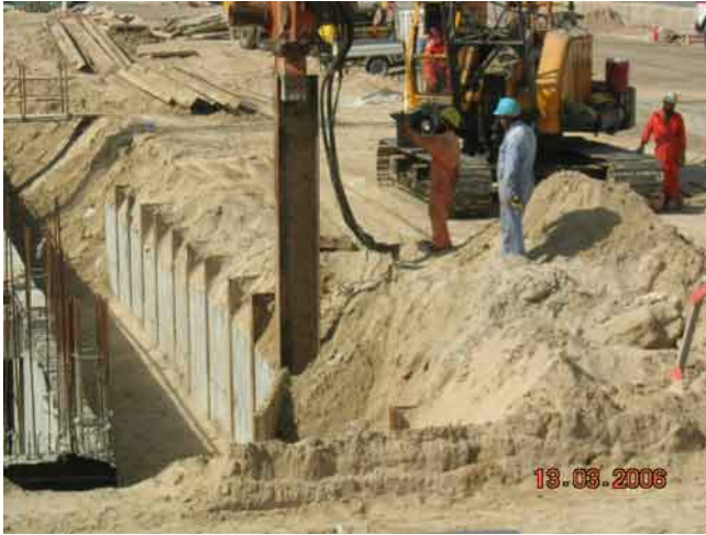
H-beams removal for parking area
