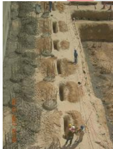
Cathodic Protection Wind Tower I
