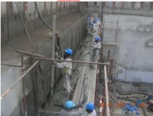
Plastering Wind Tower I
