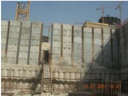
Plastering Wind Tower II
