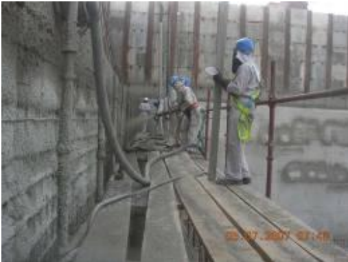
Plastering Wind Tower I
