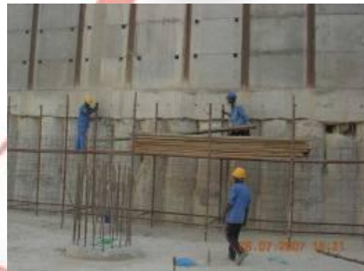
Plastering Wind Tower II
