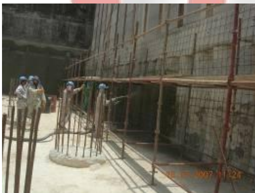
Plastering Wind Tower II
