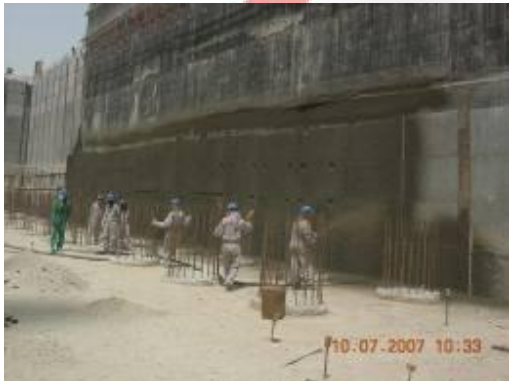
Plastering Wind Tower II
