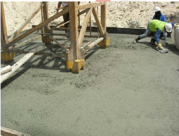
Casting for Wind Tower II
