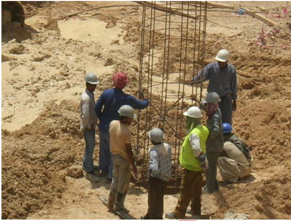
Reinforcement for Wind Tower I
