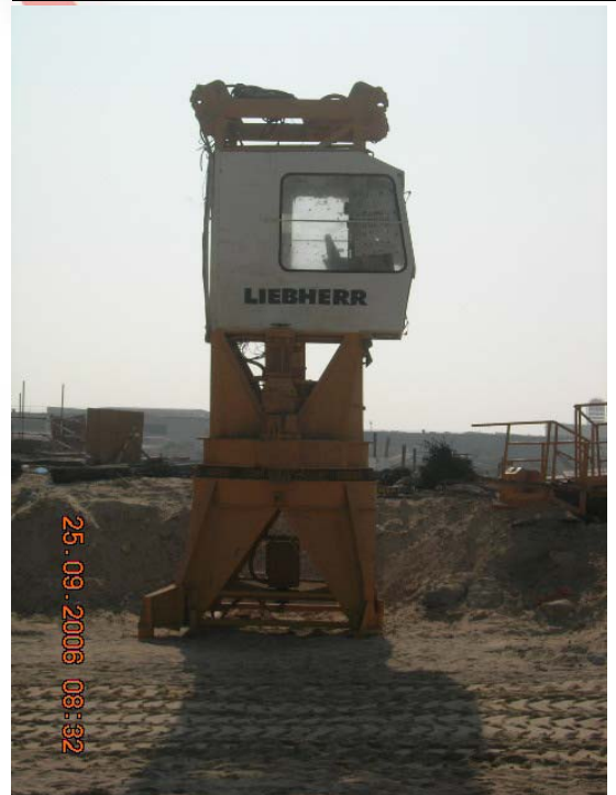
Tower Crane Erection for Wind Tower II
