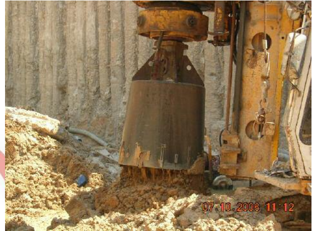
Drilling for Wind Tower I
