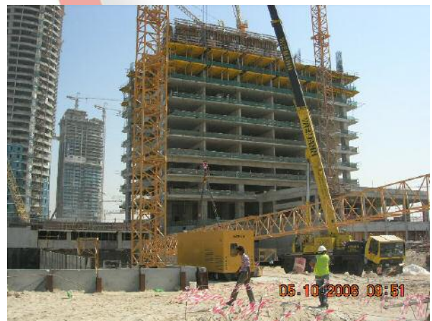
Tower Crane Erection for Wind Tower II
