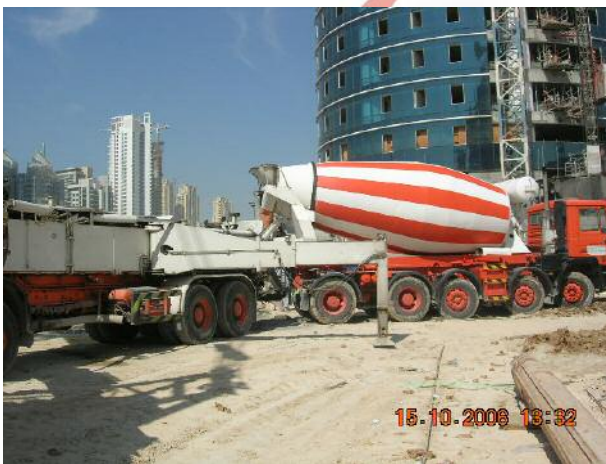
Casting for Wind Tower I
