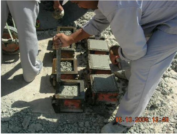
Concrete Test for Wind Tower I
