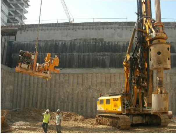
Drilling for Wind Tower I
