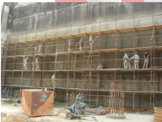
Plastering Wind Tower I
