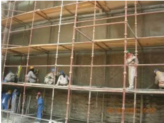
Plastering Wind Tower I
