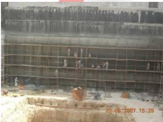
Plastering Wind Tower I
