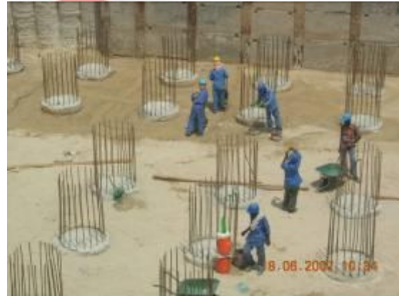
Soil Compaction Wind Tower II
