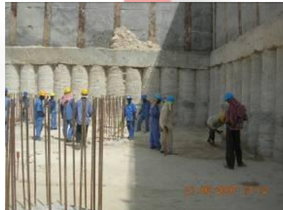
Soil Compaction Wind Tower II
