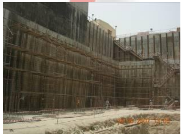
Plastering Wind Tower I
