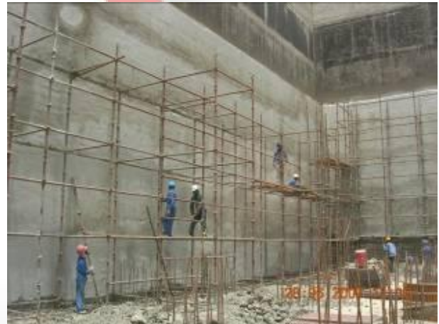
Plastering Wind Tower I
