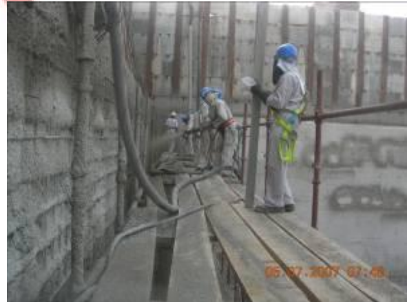
Plastering Wind Tower I
