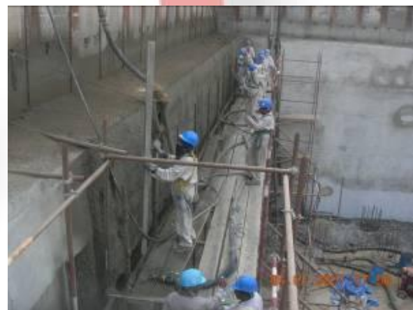
Plastering Wind Tower I
