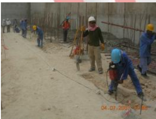
Cathodic Protection Wind Tower I
