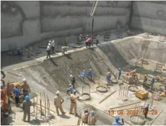
Water proofing Wind Tower I
