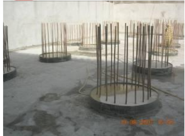
Waterproofing Wind Tower II
