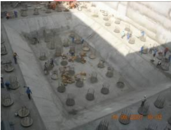
Waterproofing Wind Tower I
