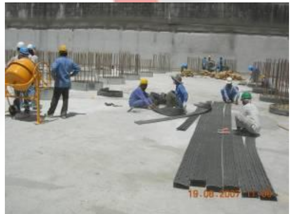
Waterproofing Wind Tower II
