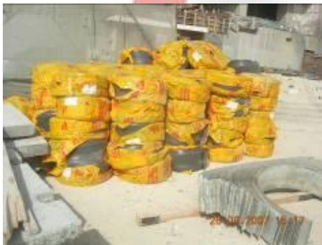
Materials arrived for water proofing
