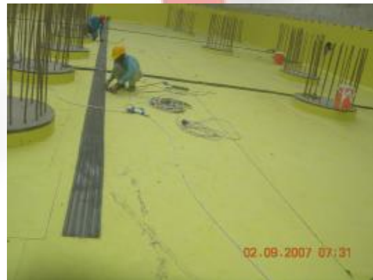
Fitting the yellow membrane with water bars Wind Tower II
