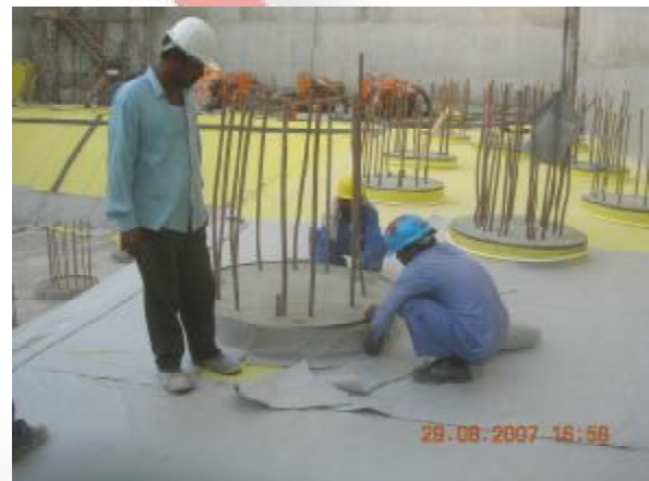
Placement of the grey membrane Wind Tower I
