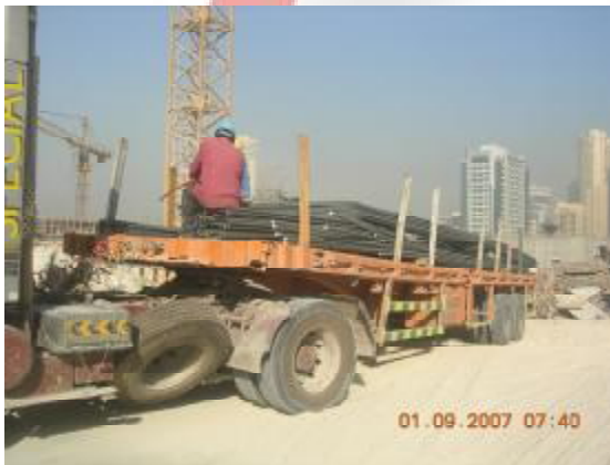
Steel bars arrived at Wind Tower I
