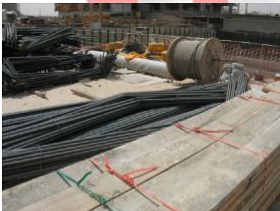
Steel bars arrived at Wind Tower I
