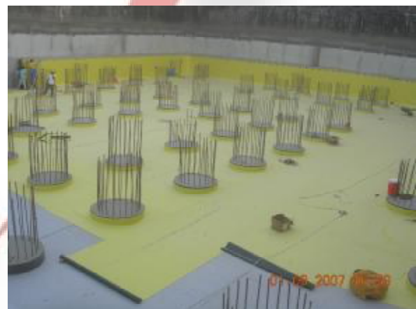
Placement of the yellow membrane Wind Tower II
