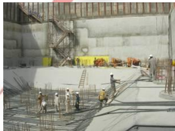
Reinforcement Wind Tower I
