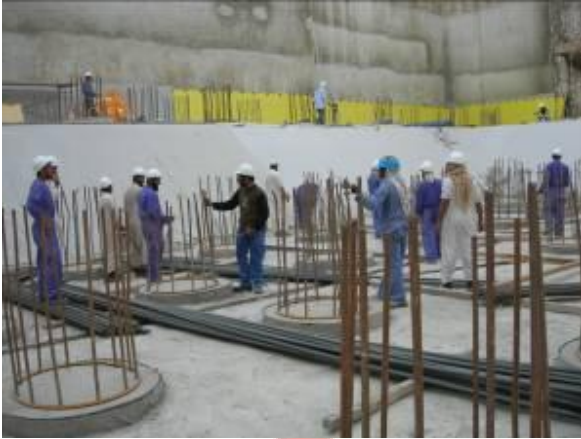
Reinforcement Wind Tower I
