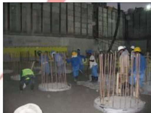
Water Proofing Wind Tower II
