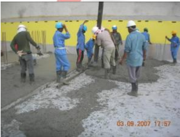
Waterproofing Wind Tower II
