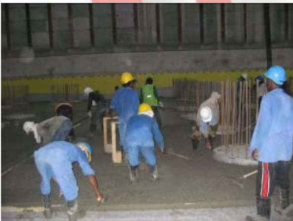
Waterproofing Wind Tower II
