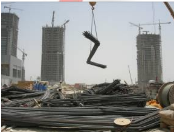
Material received for reinforcement Wind Tower I
