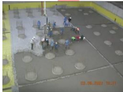
Water Proofing Wind Tower II
