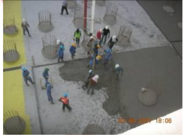
Waterproofing Wind Tower II
