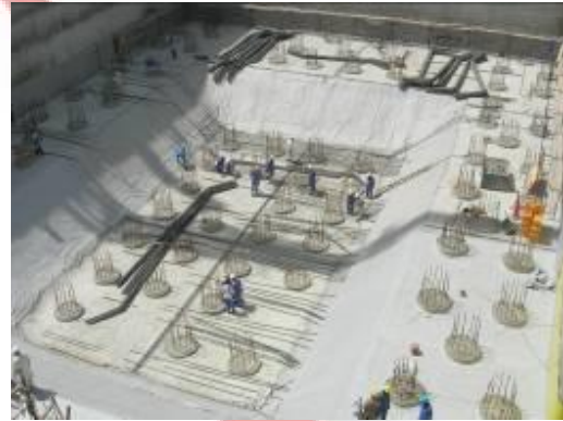
Reinforcement Wind Tower I
