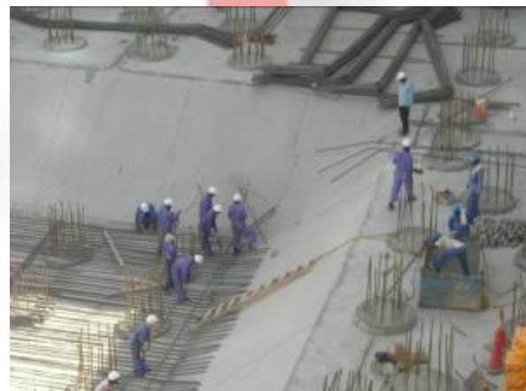
Reinforcement Wind Tower I
