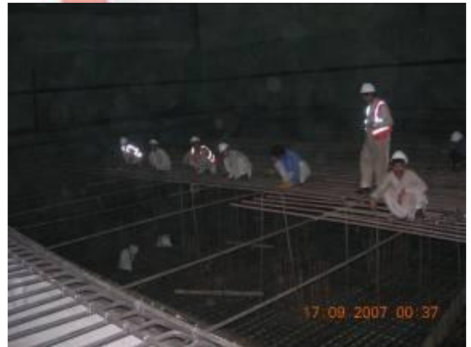
Reinforcement Wind Tower I
