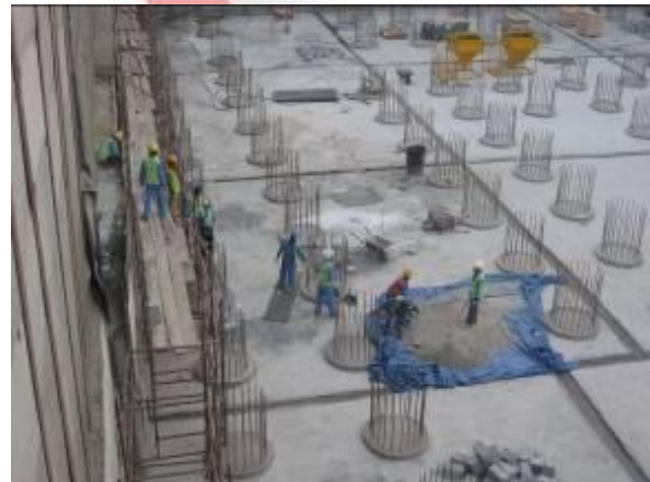
Vertical Water Proofing Wind Tower II
