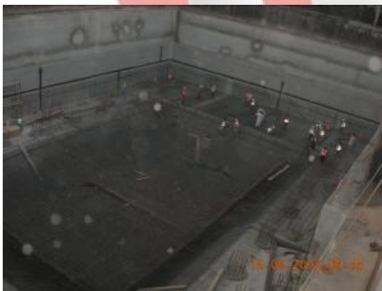
Reinforcement Wind Tower I
