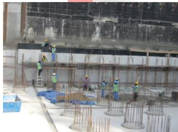
Vertical Water proofing Wind Tower II
