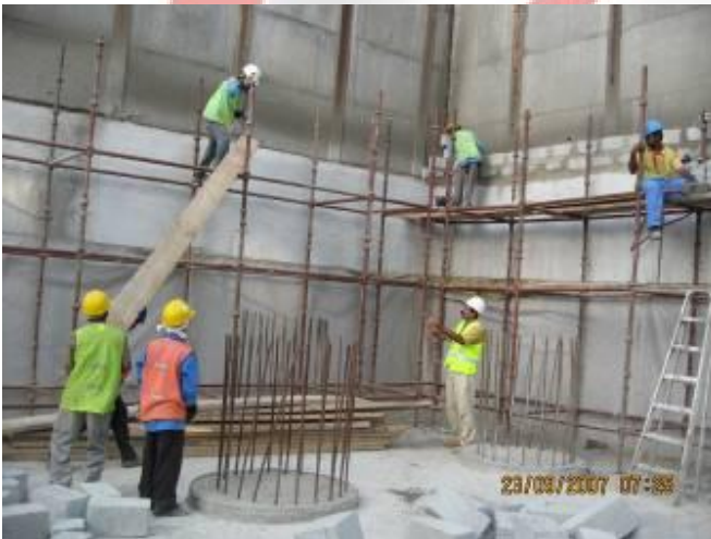
Vertical Water Proofing Wind Tower II
