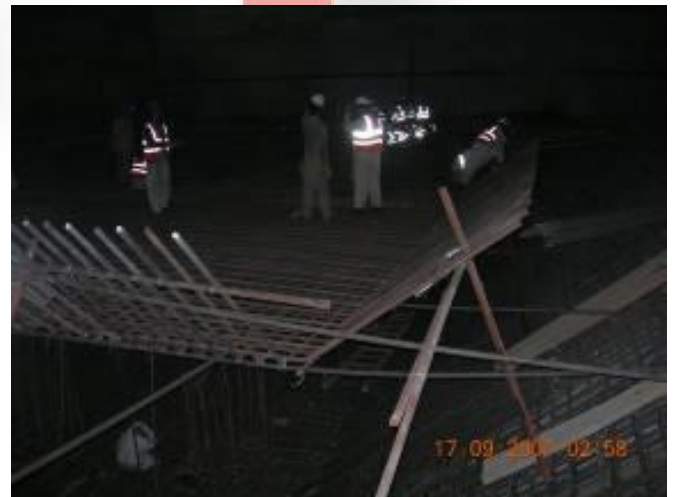
Reinforcement Wind Tower I
