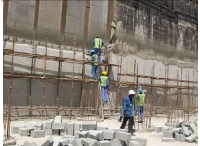
Vertical Water proofing Wind Tower II
