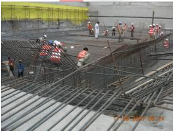
Reinforcement Wind Tower I
