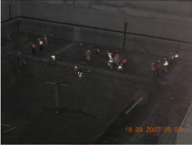
Reinforcement Wind Tower I
