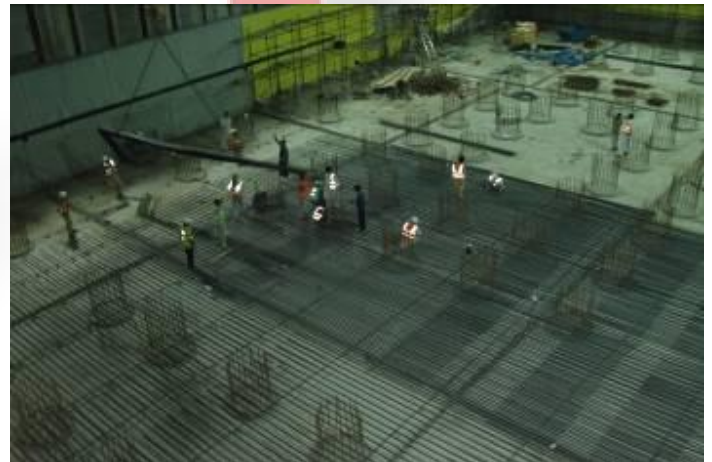
Reinforcement Wind Tower II
