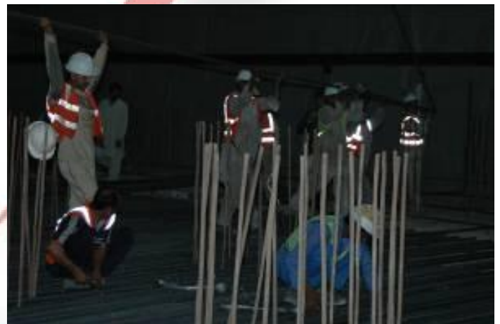
Reinforcement Wind Tower II
