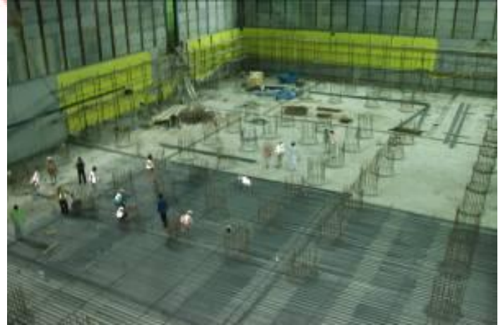
Reinforcement Wind Tower II
