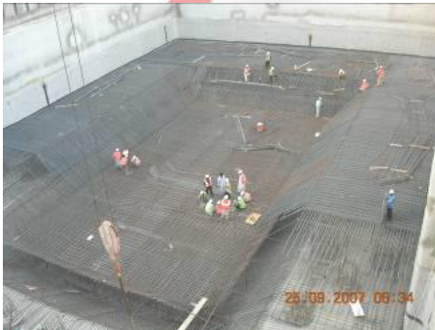
Reinforcement Wind Tower I
