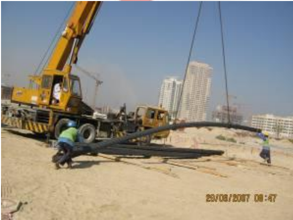
Materials Received Wind Tower II
