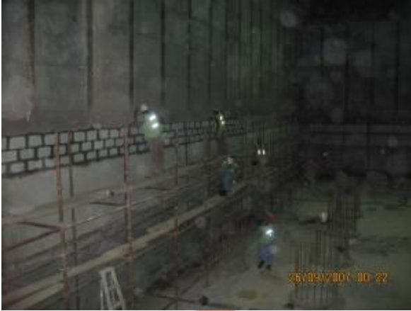
Water Proofing Wind tower II
