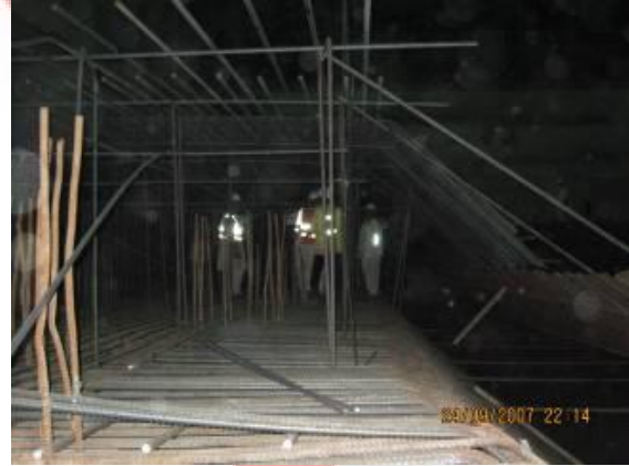
Reinforcement Wind Tower I
