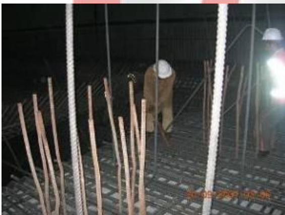
Reinforcement Wind Tower I
