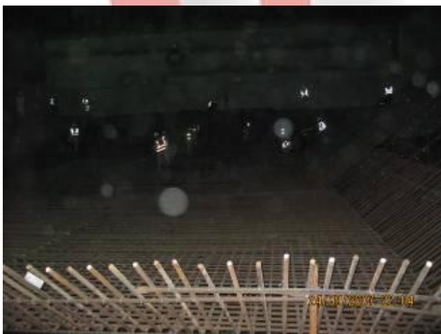
Reinforcement Wind Tower I
