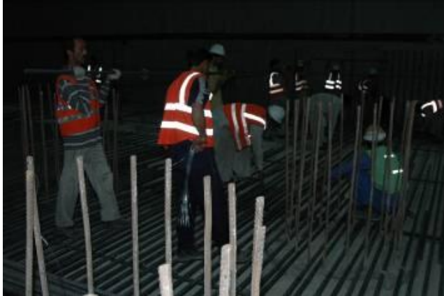
Reinforcement Wind tower II
