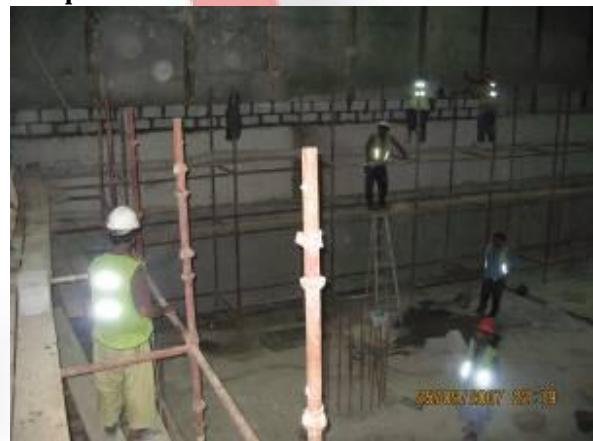
Water Proofing Wind Tower II
