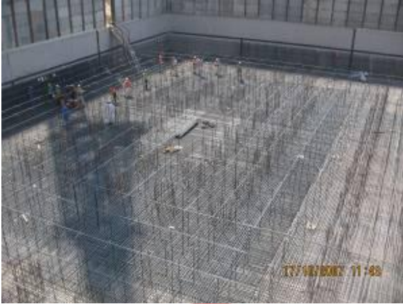
Reinforcement Wind Tower II
