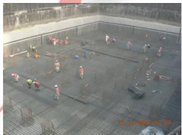
Reinforcement Wind Tower II
