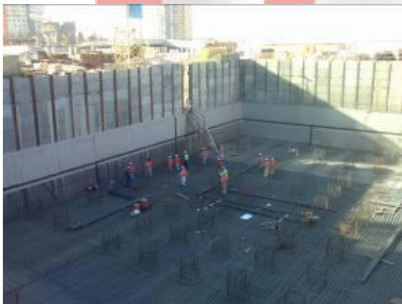
Reinforcement Wind Tower II
