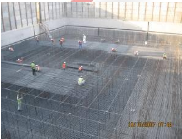
Reinforcement Wind Tower II
