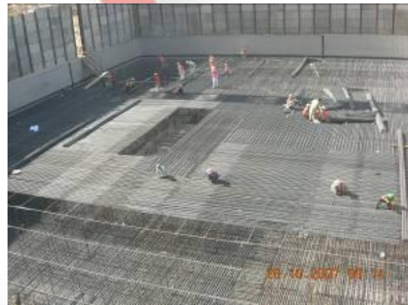
Reinforcement Wind Tower II
