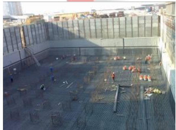
Reinforcement Wind Tower II
