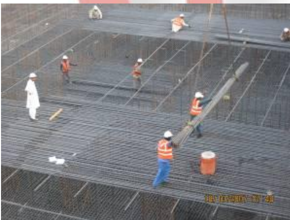
Reinforcement Wind Tower II
