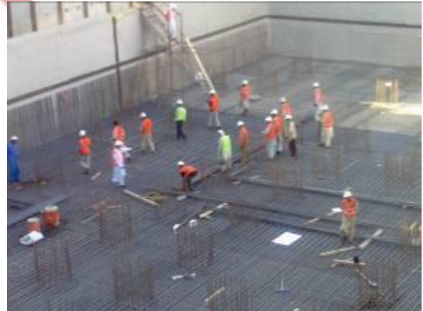
Reinforcement Wind Tower II
