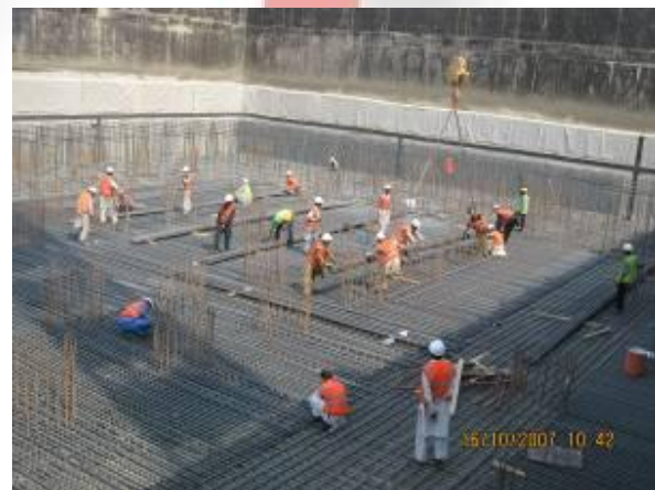
Reinforcement Wind Tower II
