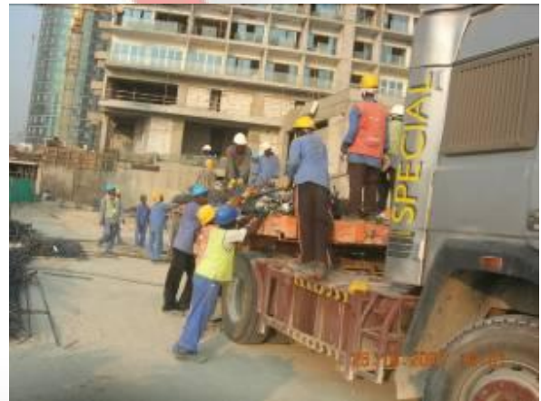
Material Received for reinforcement Wind Tower II
