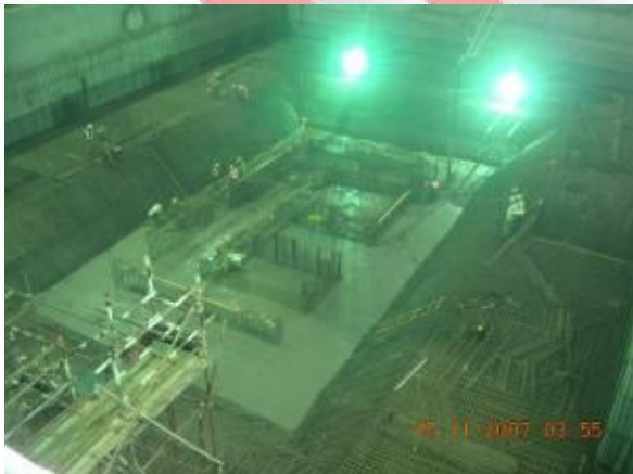
Concrete Pouring Wind Tower I
