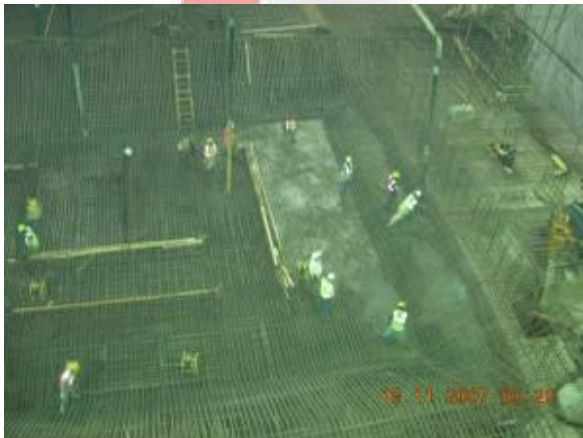
Concrete Pouring Wind Tower I
