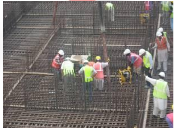
Concrete Pouring Wind Tower I
