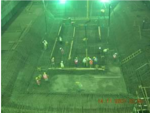
Concrete Pouring Wind Tower I
