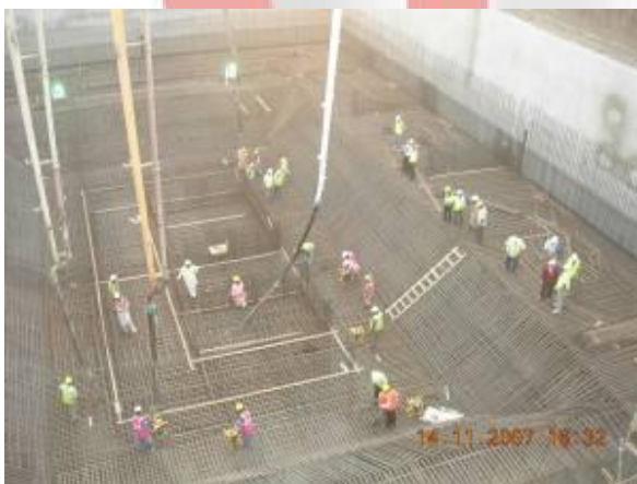
Concrete Pouring Wind Tower I
