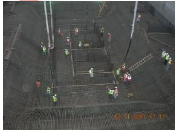
Concrete Pouring Wind Tower I
