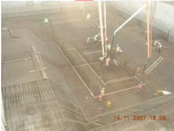
Concrete Pouring Wind Tower I
