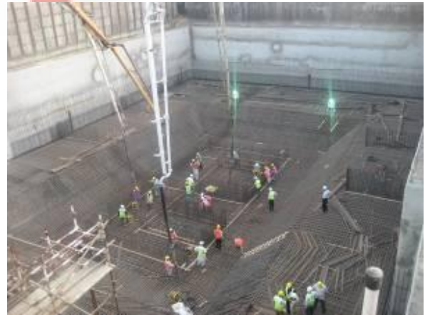
Concrete Pouring Wind Tower I
