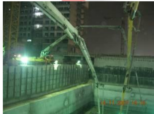
Concrete Pouring Wind Tower I
