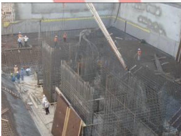
Concrete casting at the Central Core Wind Tower I http://www.faravand.org/wind%20process/process%20page.htm
