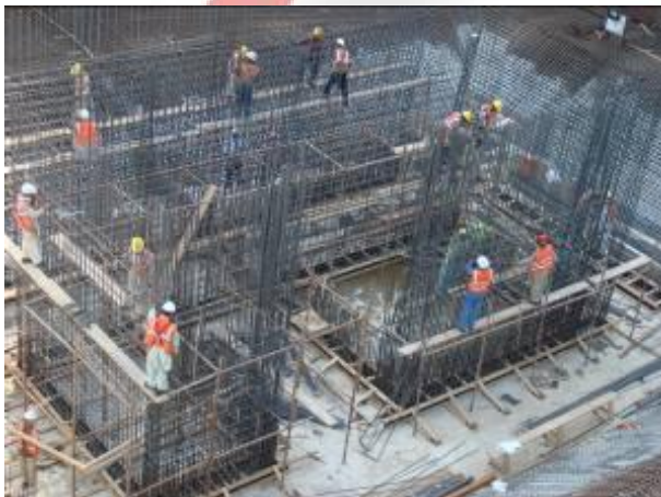
Central Core Reinforcement Wind Tower I
