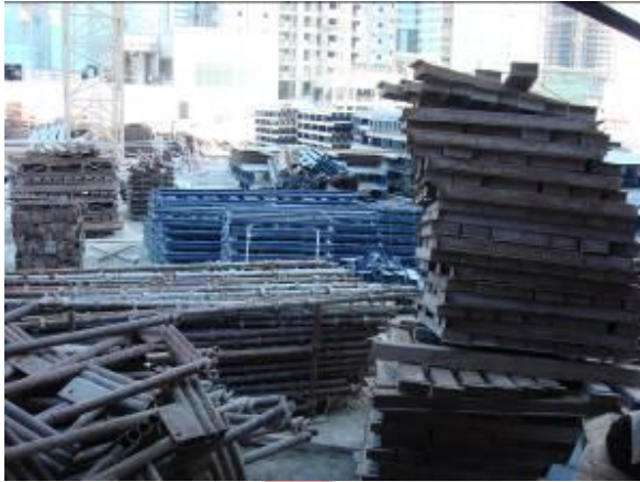
Reinforcement, casting & Shuttering Material Wind Tower I & II
