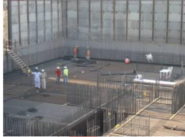
Reinforcement Wind Tower II
