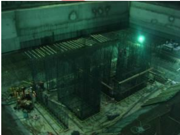
Night shift reinforcement Wind Tower I
