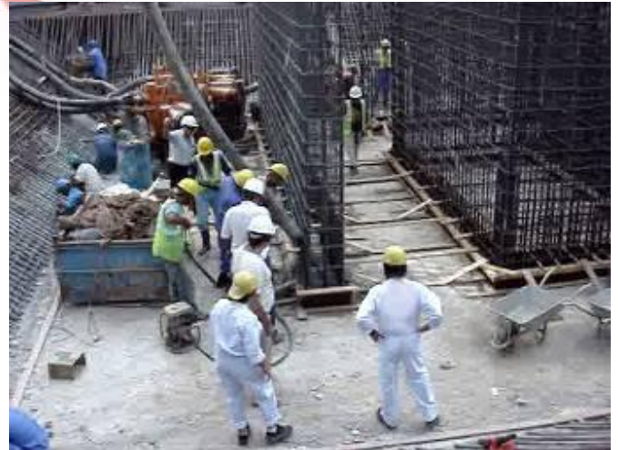
Central core concrete casting Wind Tower I
