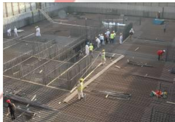
Final part of reinforcement Wind Tower II
