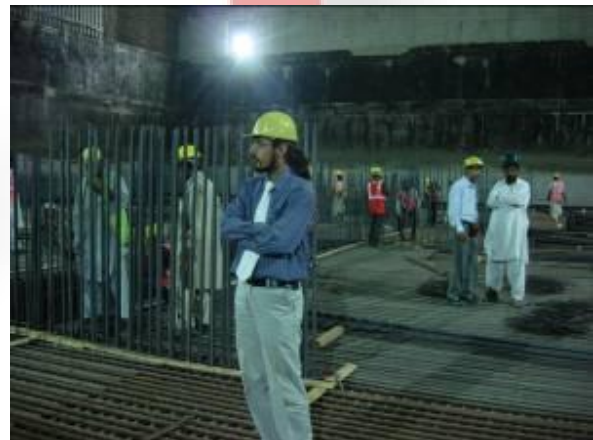
Night shift reinforcement Wind Tower II
