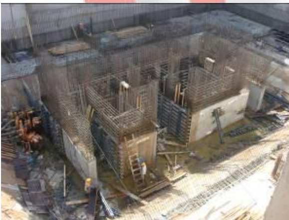
Shuttering of Wind Tower I
