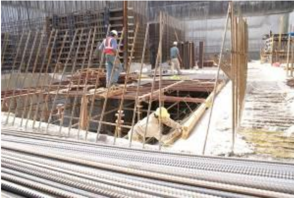
End stage of shuttering of Wind Tower I
