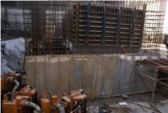
Central core shuttering of Wind Tower I
