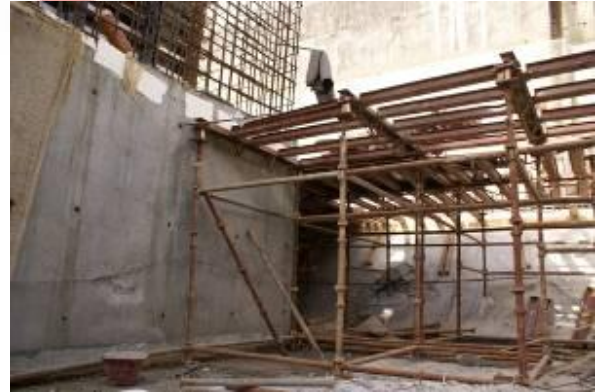
End of basement 6 of Wind Tower I
