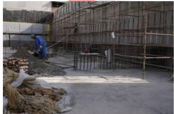
Plastering & water proofing of Wind Tower II
