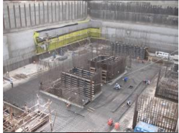
Wind Tower I
