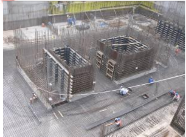
Fixing of reinforcement bar for B5 Wind Tower I
