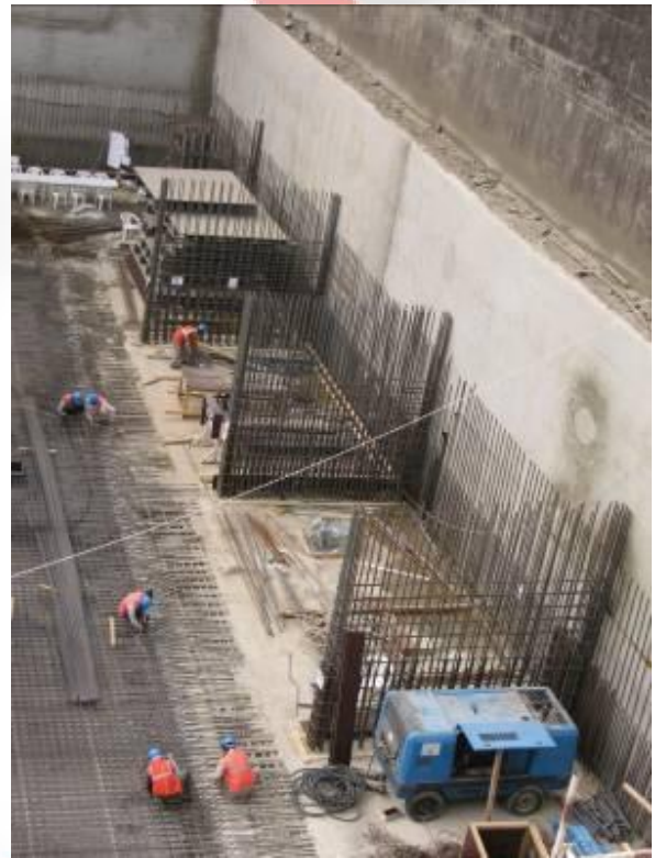
Wind Tower I
