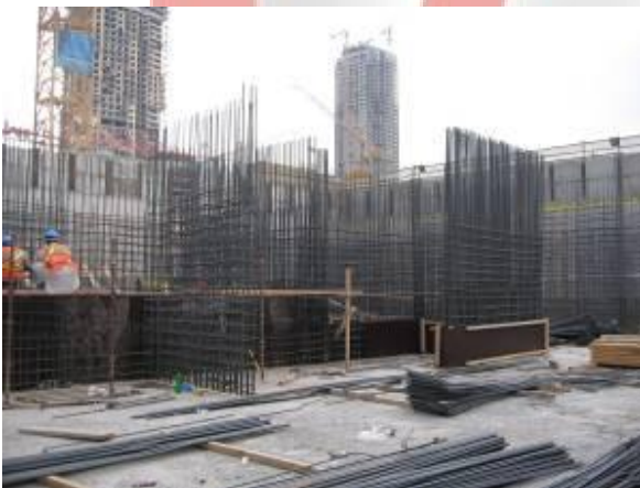
Shuttering Wind Tower II
