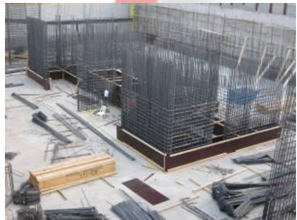
Steel bar fixing of main core Wind Tower II
