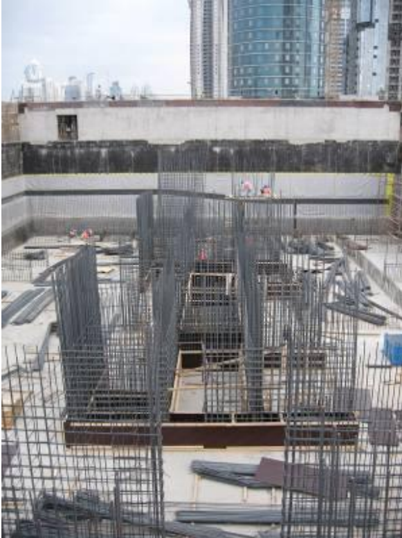
Main core steel bar fixing Wind Tower II
