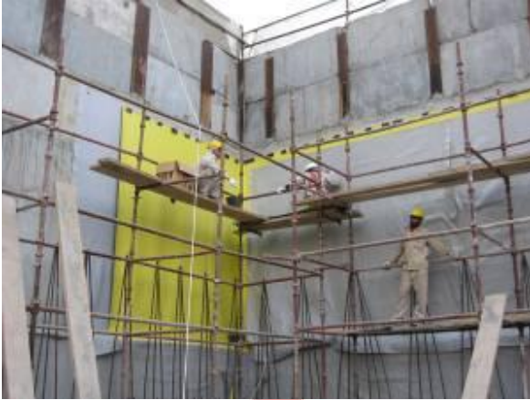
Water proofing Wind Tower II
