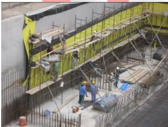
Water proofing of the wall Wind Tower I
