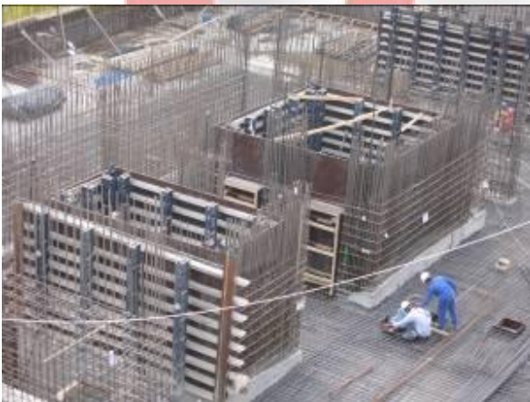
Completion of shuttering Wind Tower I
