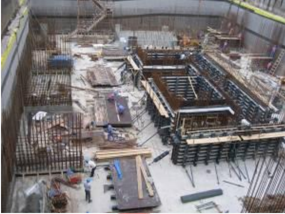
Preparing for casting in Wind Tower I
