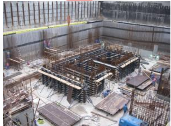
Wind Tower I after kickers Casting
