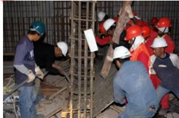
Kickers casting Wind Tower I
