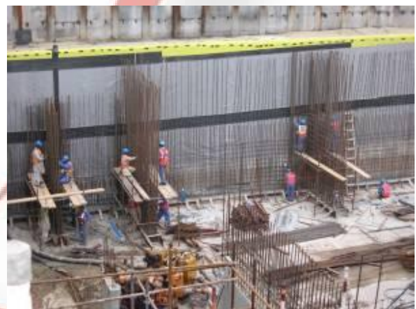
Reinforcement bar fixing of vertical elements in Wind Tower I
