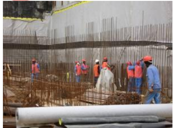
Wind Tower II
