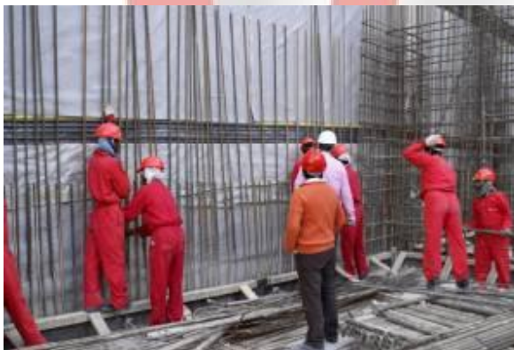
Steel bar installation for retaining wall Wind Tower I
