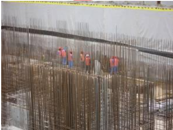
Retaining wall steel bar fixation Wind Tower II
