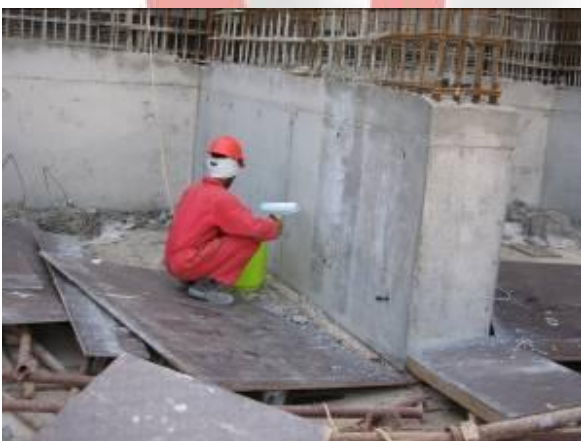
Curing of the vertical elements in Wind Tower II
