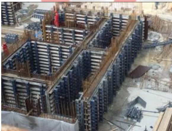
Shuttering of the main core Wind Tower I
