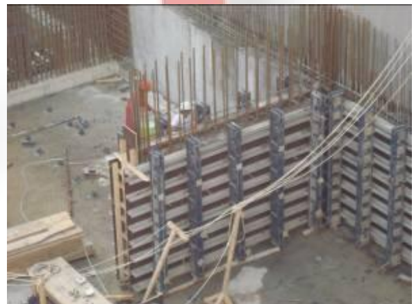
Shuttering of the vertical elements Wind Tower I
