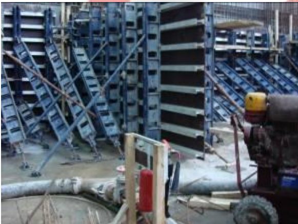
Shuttering of remaining retaining wall Wind Tower I
