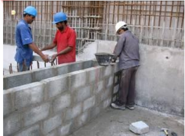
Shuttering of the water tank in Wind Tower II
