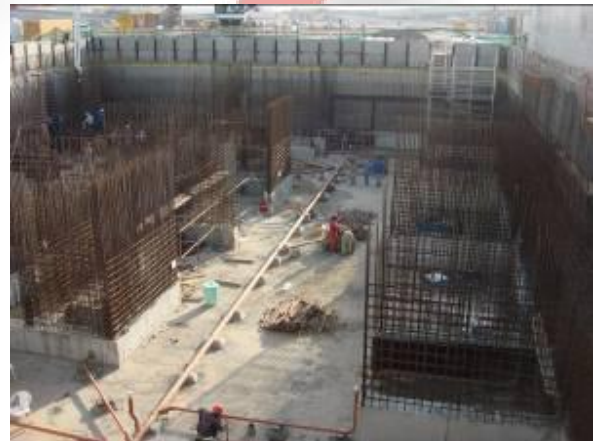
Vertical elements in Wind Tower II
