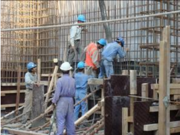
Casting of retaining wall in Wind Tower I
