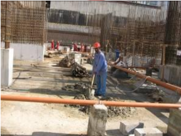
MEP work in Wind Tower II
