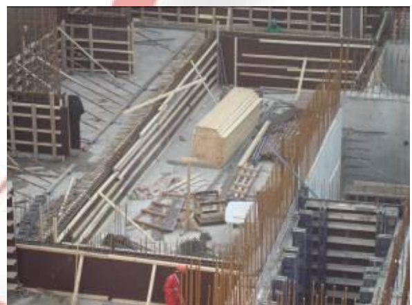
Shuttering of water tank Wind Tower I
