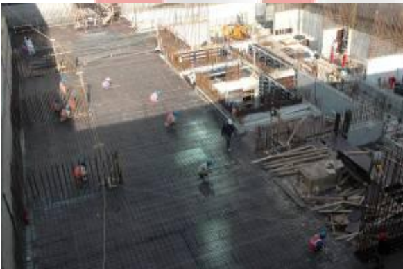
Steel bar fixing Wind Tower I
