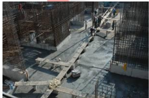
Wind Tower II casting
