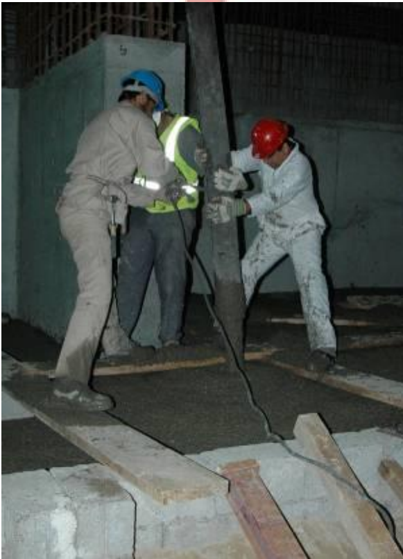
Night shift casting Wind Tower I
