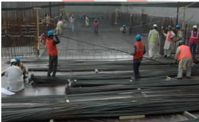
Steel bar fixing for B4 Wind Tower I
