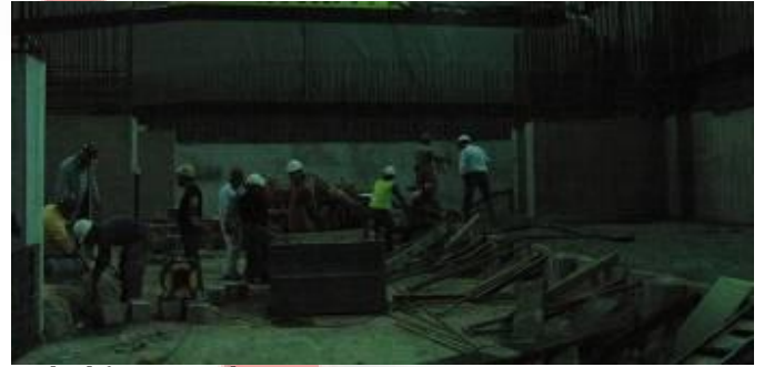
Night Shift casting Wind Tower I
