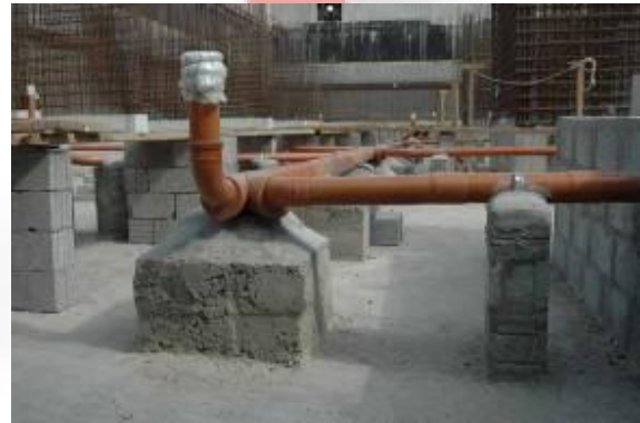
MEP work in Wind Tower II
