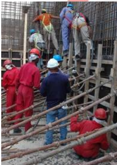
Casting of Retaining Wall Wind Tower I
