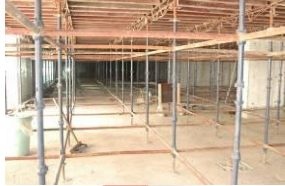
Scaffolding of the B4 Wind Tower I
