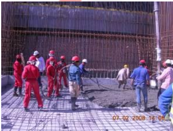
Casting of the Ramp Wind Tower II
