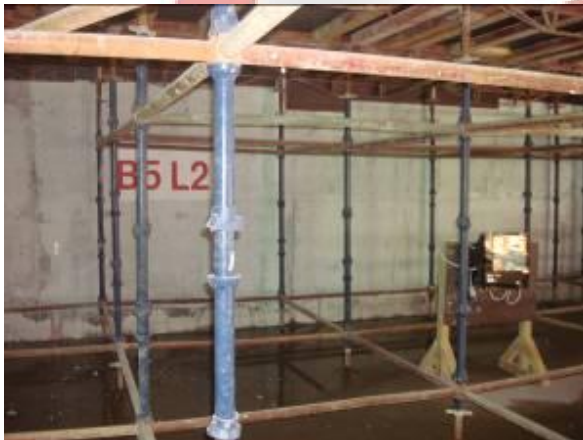
Scaffolding of L2B5, Wind Tower I
