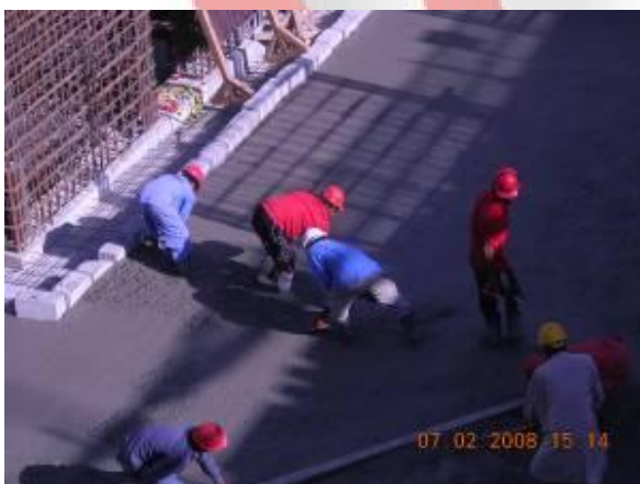
Leveling of Wind Tower II
