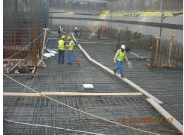
B3, Wind Tower I
