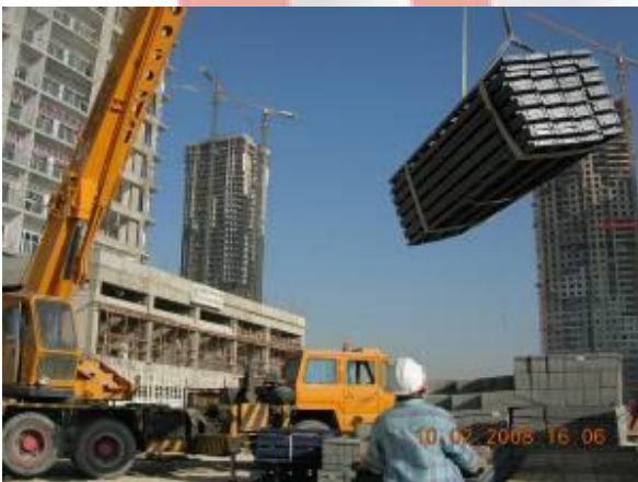
Shutters arriving to the construction site
