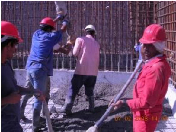
Casting in Wind Tower II
