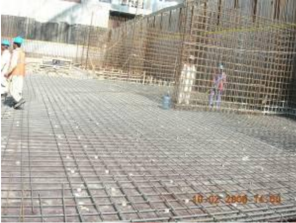
Preparing Wind I for Casting of B3
