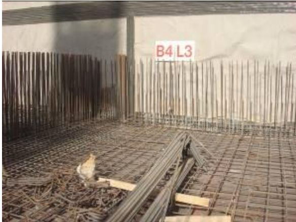
Preparing for casting of B4L3, Wind Tower I
