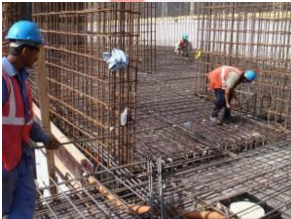
Steel bar fixing in Wind Tower I
