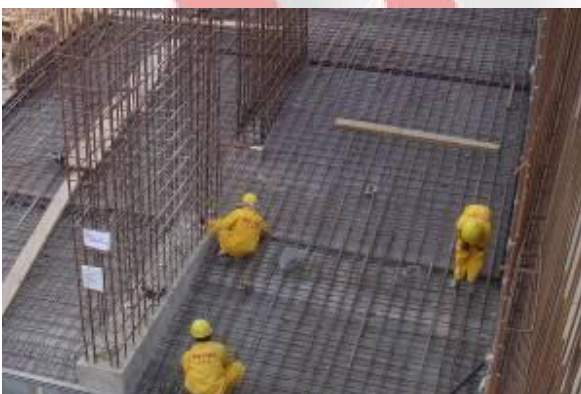
Reinforcement bar fixing in Wind Tower II
