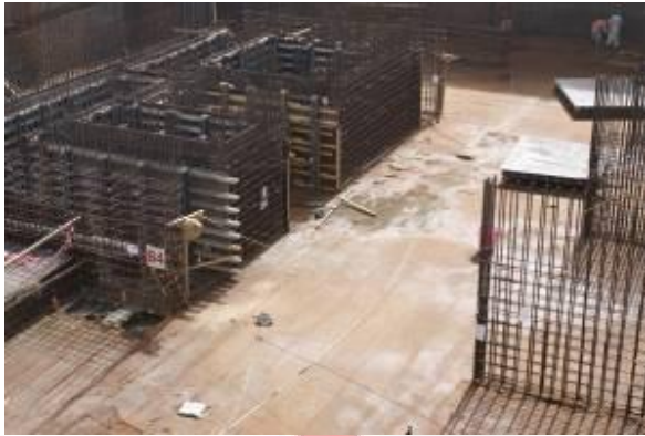
Curing of L3 Wind Tower I
