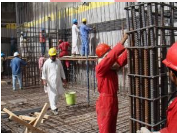
Steel Bar fixing in Wind Tower II
