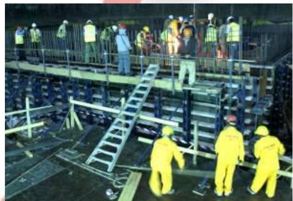
Casting of the main core in Wind Tower I
