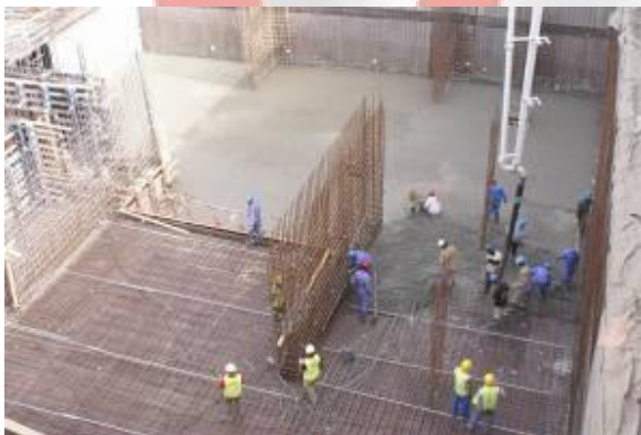
Casting of L3 Wind Tower I
