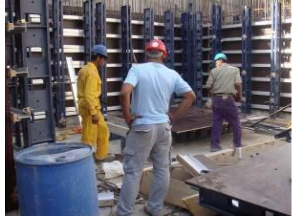
Shuttering of vertical elements in Wind Tower II
