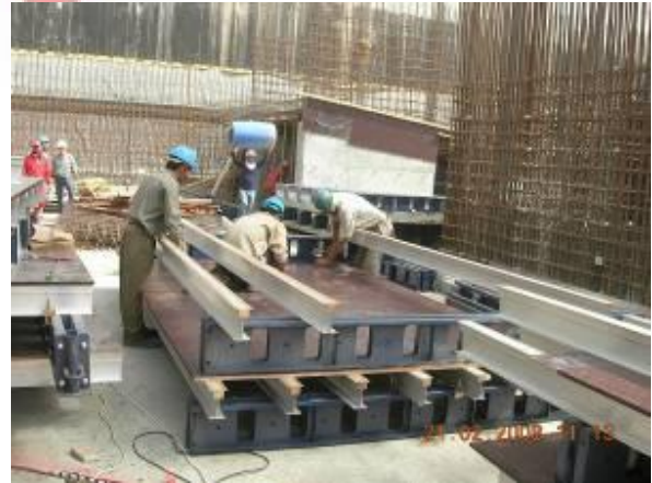
Shutters of Wind Tower II
