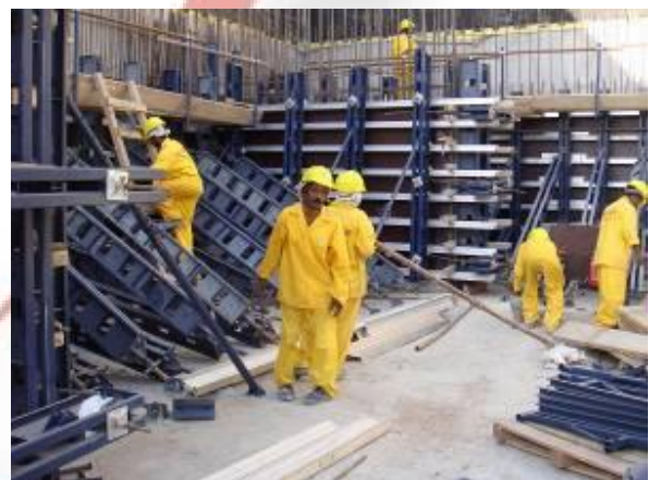
Work progress in Wind Tower II
