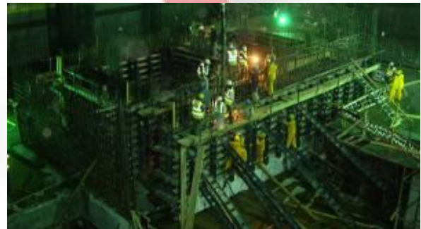
Casting of the main core in Wind Tower I
