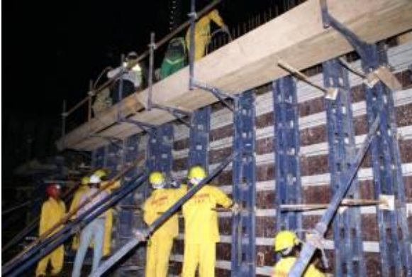
Night Shift work in Wind Tower I
