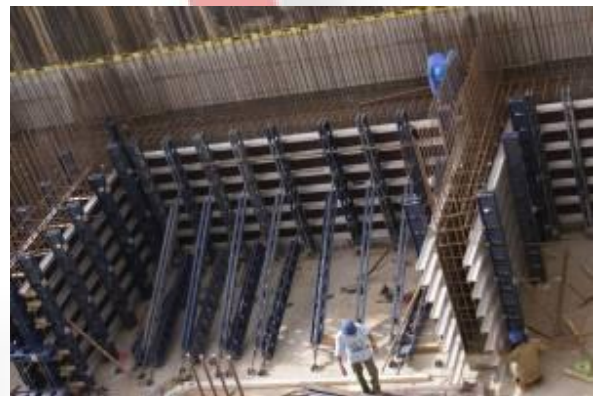
Shuttering of Wind Tower II
