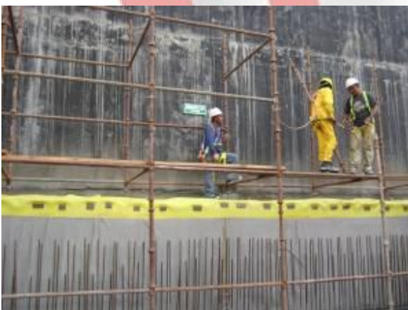
Scaffolding installation Wind Tower I
