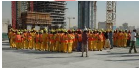
New labors for Wind Tower I & II
