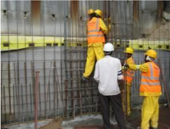
Column re-enforcement fixing Wind Tower I
