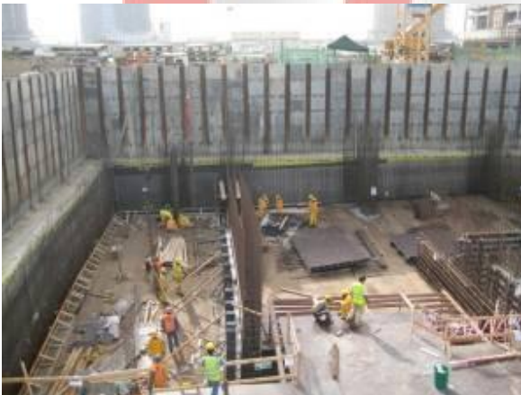
Kicker Shuttering of L3-L2 Wind Tower I
