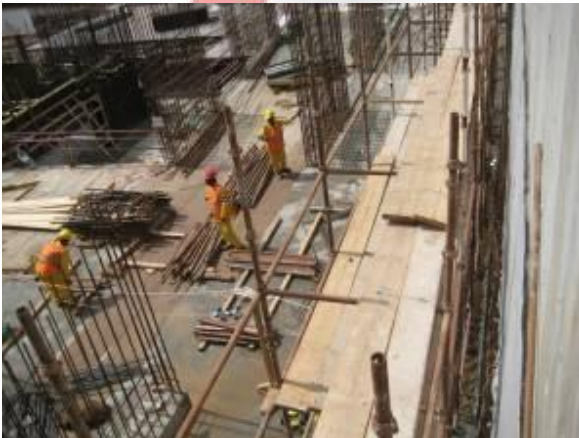
Column re-enforcement fixing Wind Tower I
