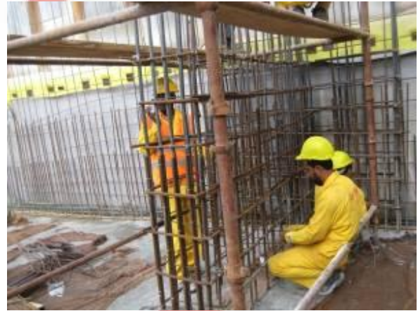
Column re-enforcement fixing Wind Tower I
