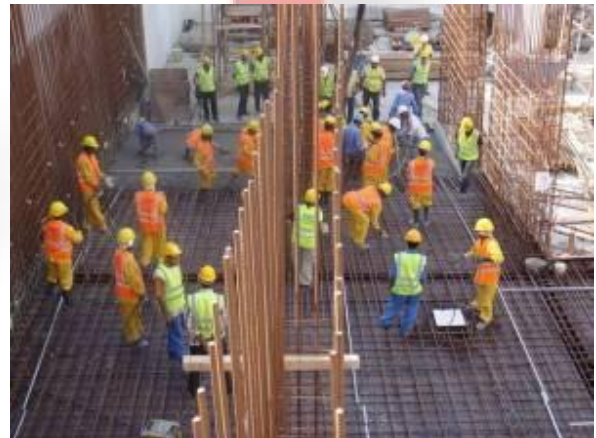
Half of L2 area casting is completed - Wind Tower II
