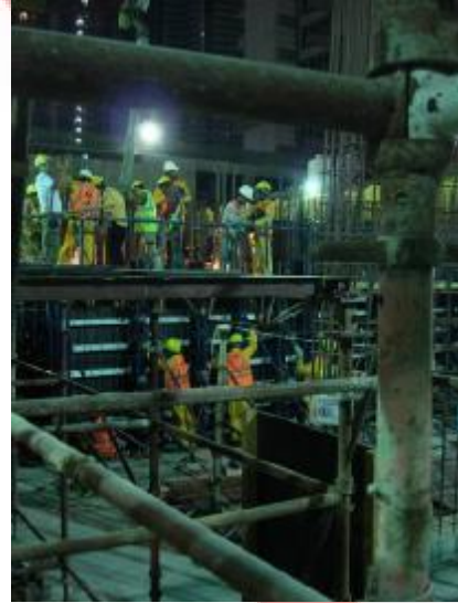
Wind Tower II
