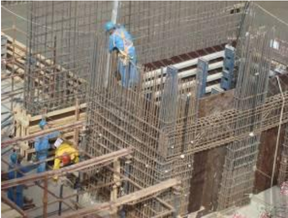
Wind Tower I
