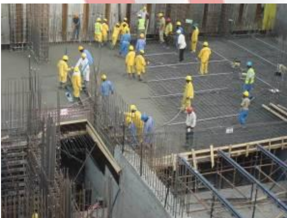
Wind Tower I
