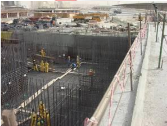
Wind Tower I
