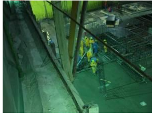
Wind Tower I
